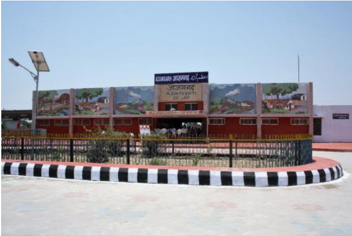
Railway station, Azamgarh
